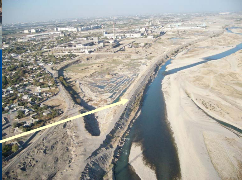
Dam for Flood Control
