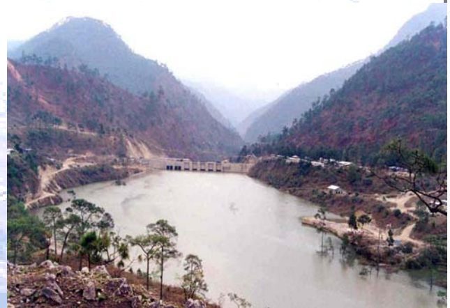
Kurichhu Hydropower Plant
