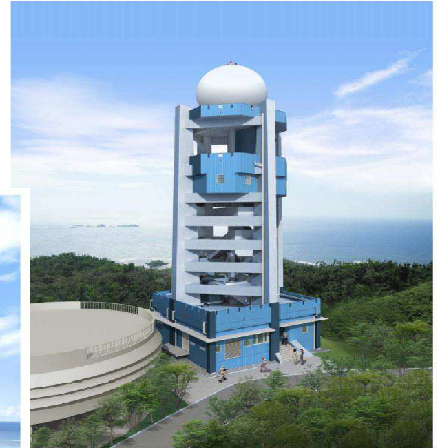
Virac Meteorological Radar Tower Building
