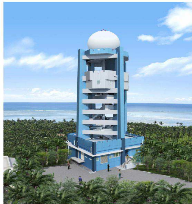
Guiuan Meteorological Radar Tower Building
