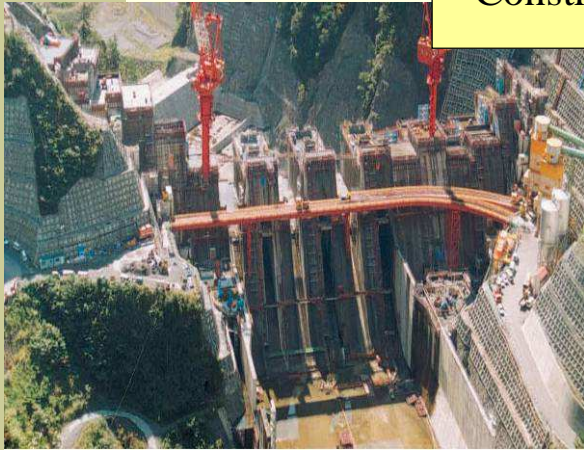
Flood control (Dam)
