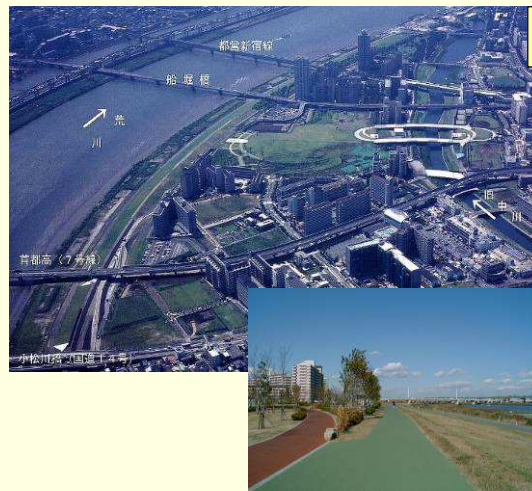
High standard embankments
