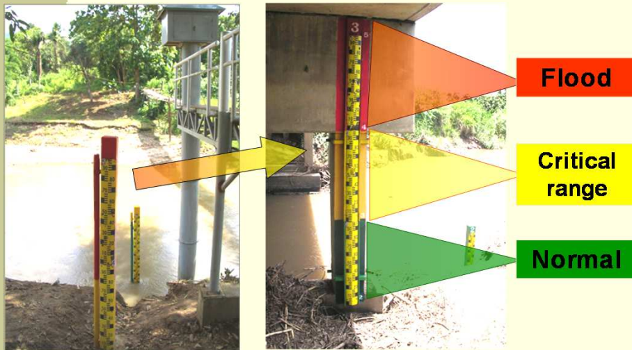
Fig.40 Colored staff gauge to easily identify flood risk (Thadu, 2009)
