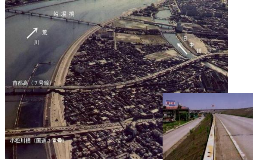
River discharge secured (Super Levee)
