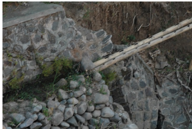
Damaged hydraulic structure by flood flow, MSB Kusuma, 2008
