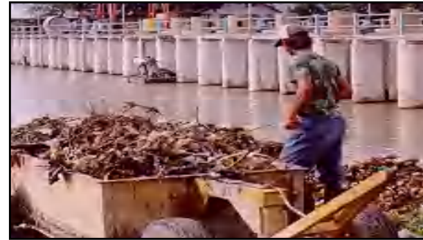
Debris in Curug Weir
