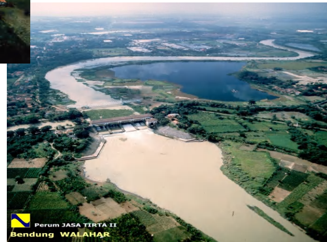
WALAHAR WEIR IN CITARUM RIVER BASIN
