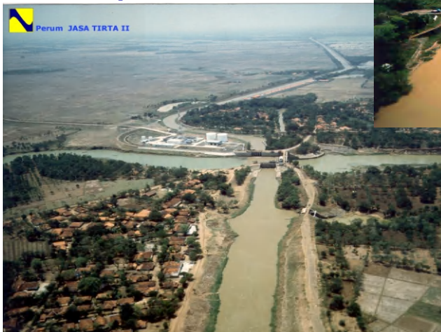
SALAM DARMA WEIR IN CIPUNEGARA RIVER Operation of 1923
