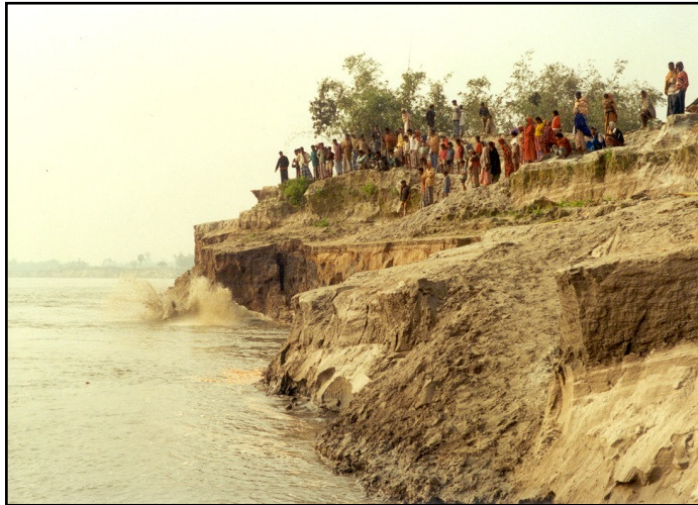
River Bank Erosion
