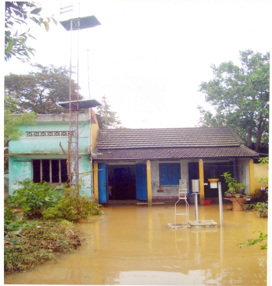
Phu Oc Station in Bo river basin in flood caused by Sangsan typhoon in 2006
