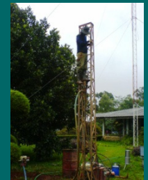
Making well at NO.4
