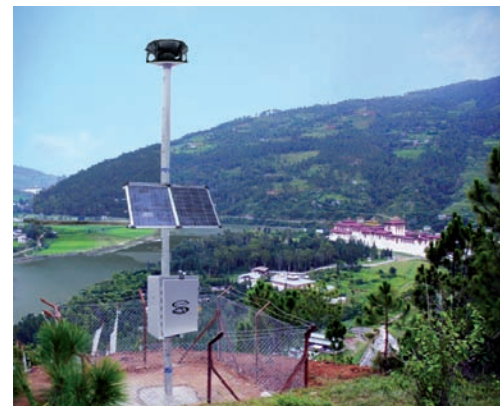
17 siren stations have been set up across the kingdom. Sirens are triggered as stream thresholds are exceeded
