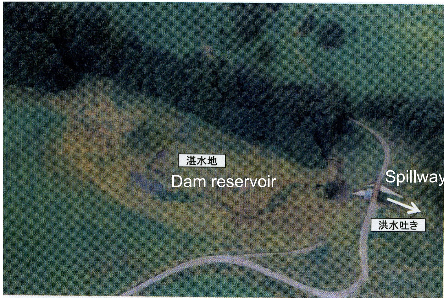
Gabriachbach Eichengrund overall view
