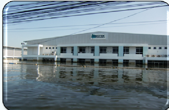
Too Much Water
